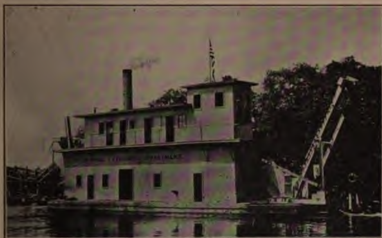
View of Excavating End of Elevator Dredge on Fox River, Wisconsin. Figure 100.
